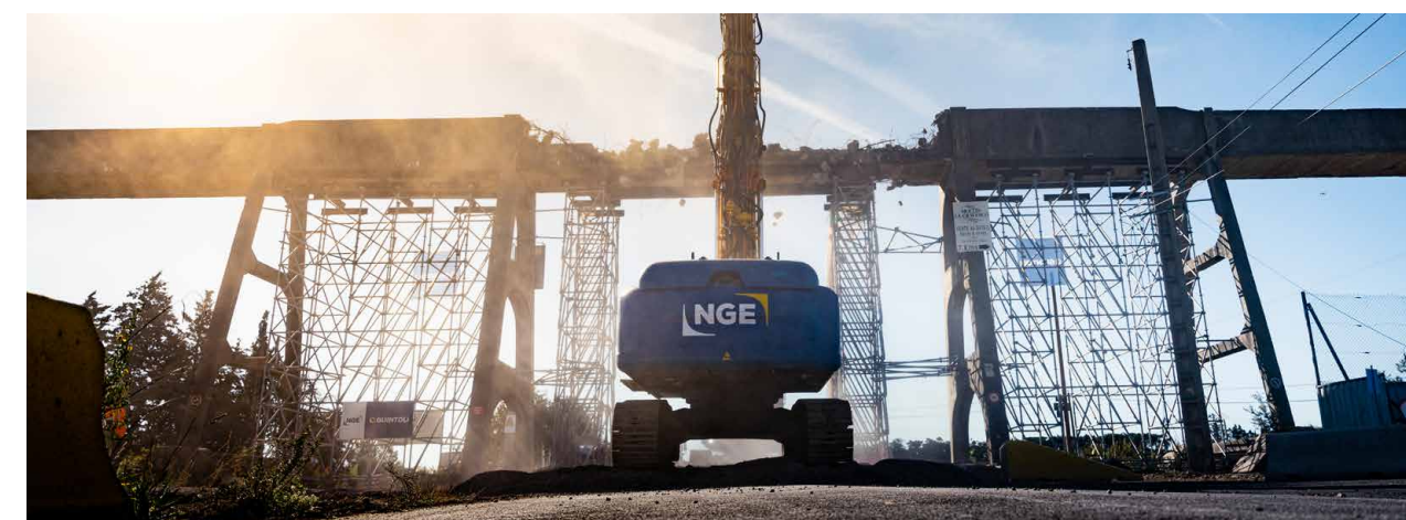
Deconstruction of the Fourbine aqueduct in Saint-Martin-de-Crau (13)
