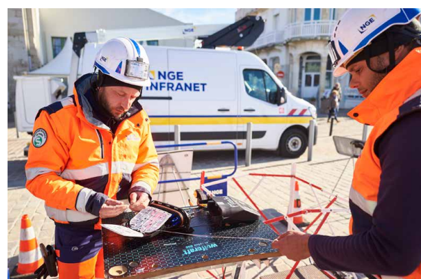
Deployment of optical fiber in Aquitaine
