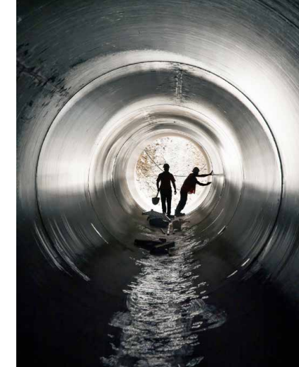
Creation of 200 linear meters water network rainwater in DN2800 in Villeneuve-les-Avignon (30)
