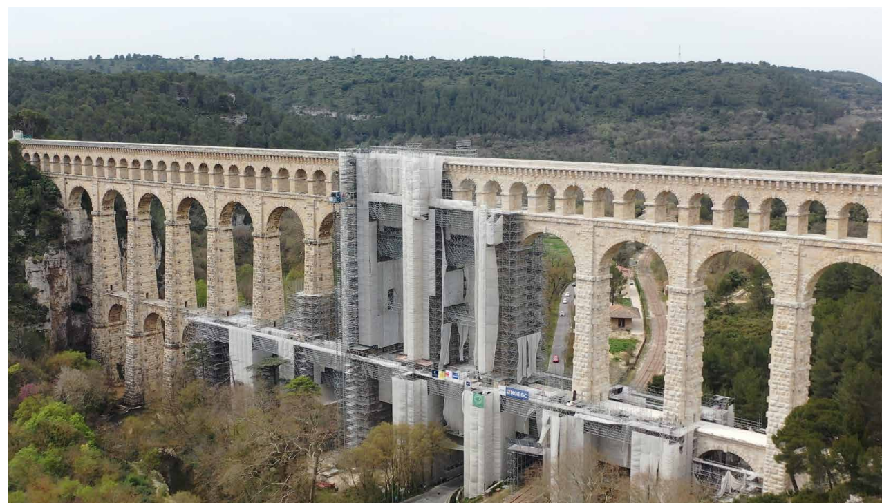
Renovation of the Roquefavour aqueduct (13)
