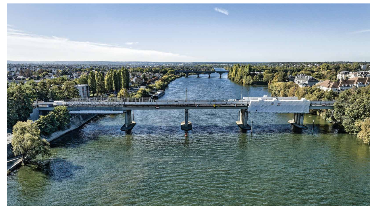
Renovation of the Maisons-Laffitte bridge (78)
