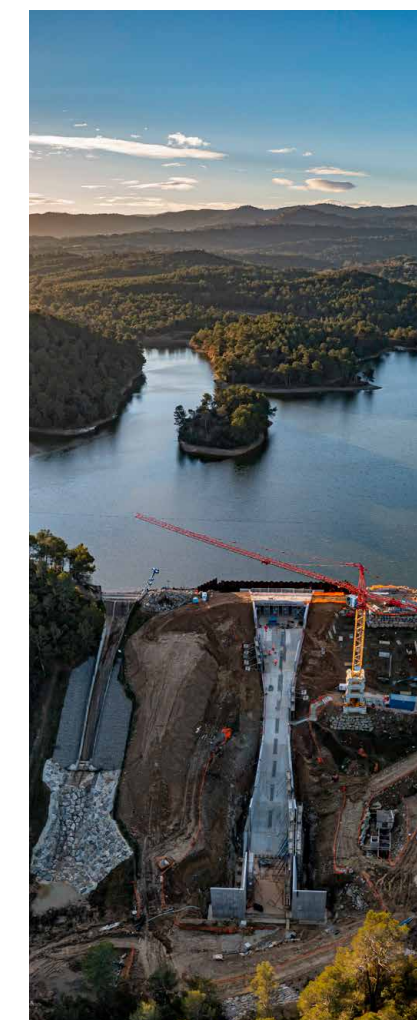
Lake security works of the Cavayere (11)
