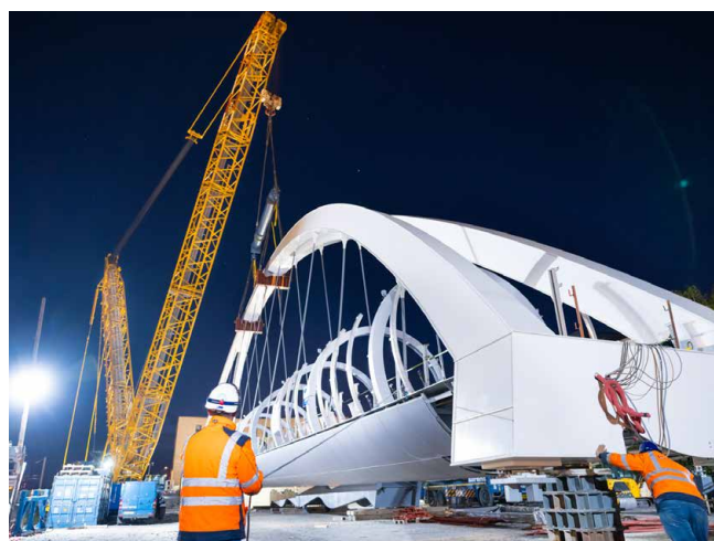
Installation of the Hazebrouck footbridge (59)
