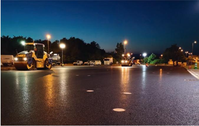
**“Together with NGE, we took the decision to carry out tests using a specially formulated asphalt surfacing mix to provide better resistance to thermal and mechanical aggression, at the same time as extending the working life of the wearing course. This approach is fully consistent with our commitment to minimising the environmental footprint of our worksites and to making the roadbuilding industry cleaner and more sustainable”.**
