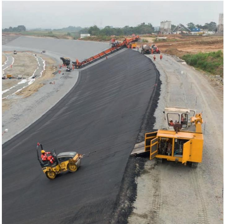
The 35-metre beam paver applies waterproof surfacing to the Nachtigal Dam power channel
