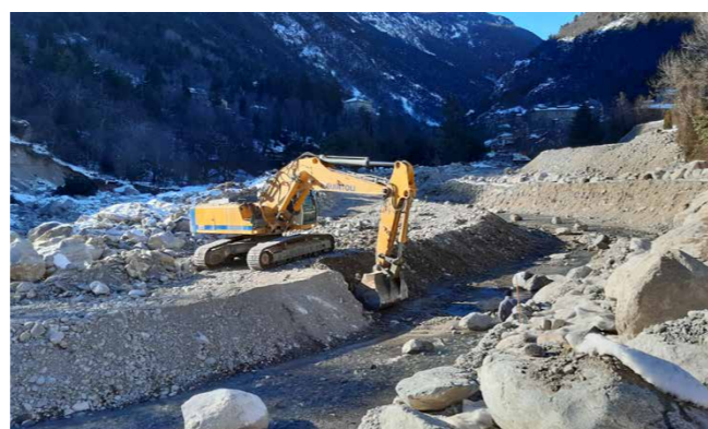
Restoration works in Middle Romansh
