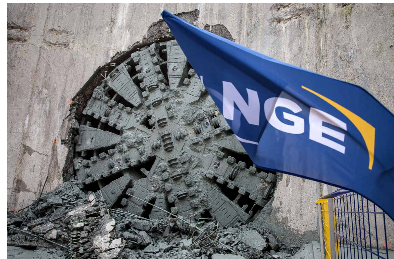
Grand Paris Express - Line 16 - Drilling of the Mireille tunnel boring machine
