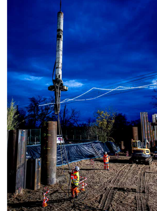
Construction site PN288
