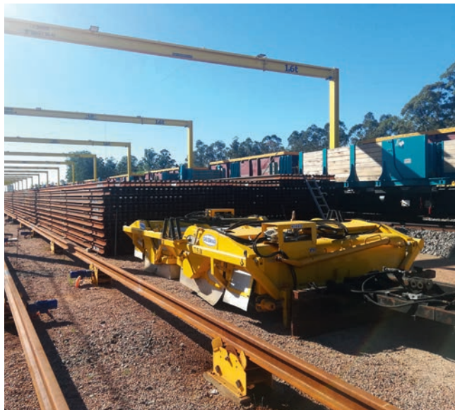
► Installing rail bridge girders and unloading machinery
