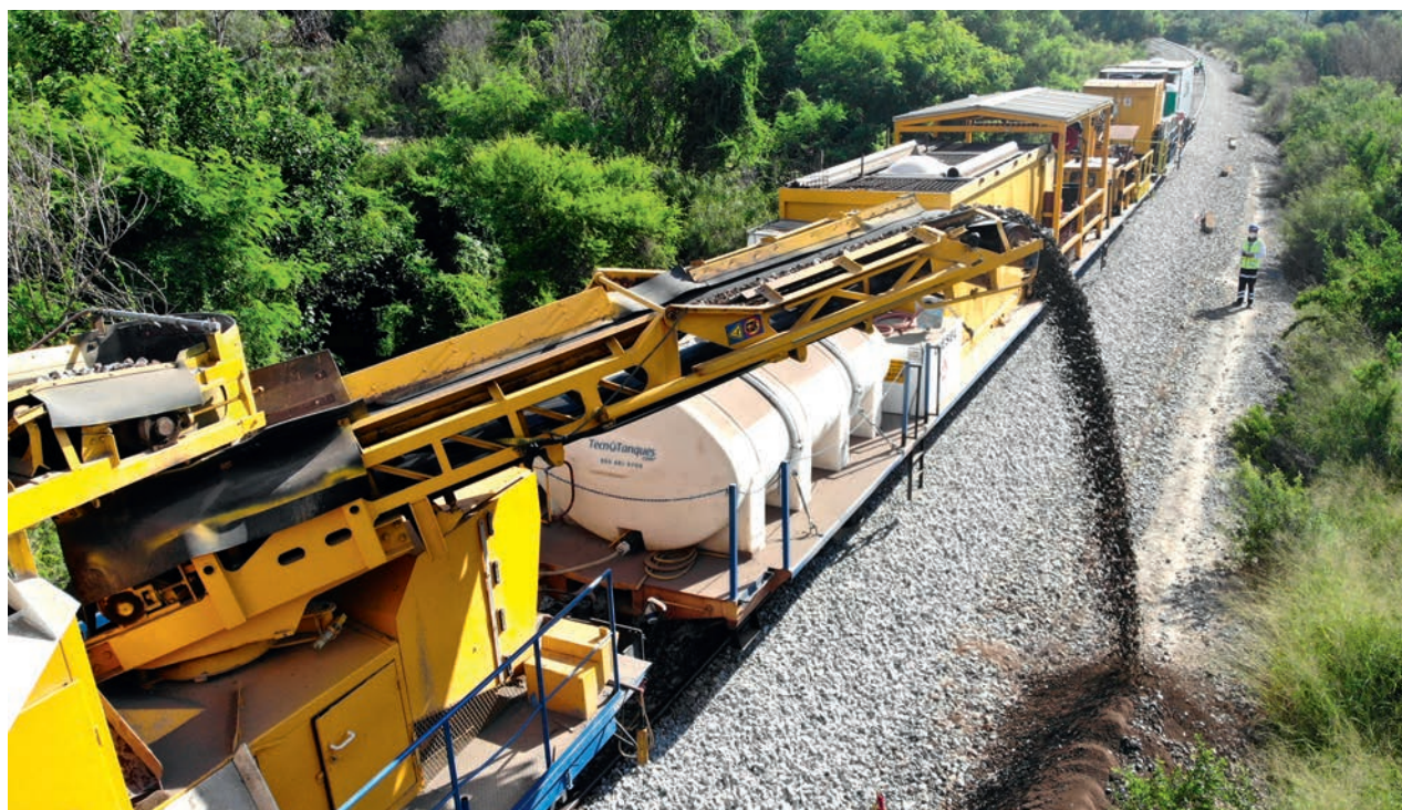
Rail contracting in Mexico
