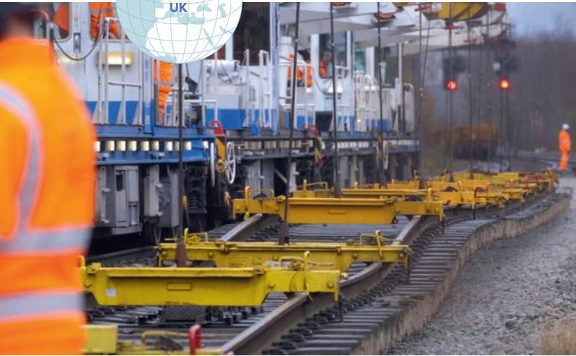
Track replacement in the UK
