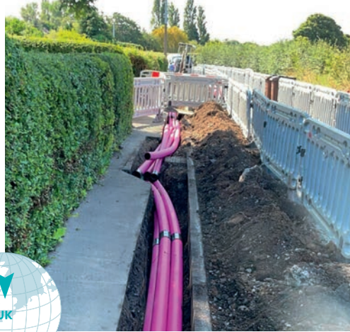
The first trenches are dug for the Liverpool optical fibre rollout
