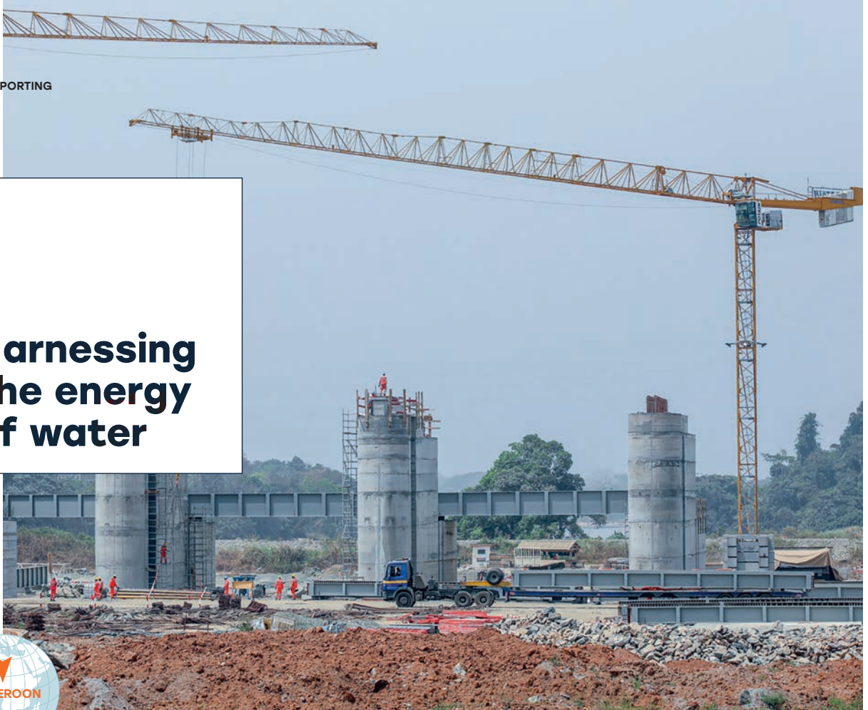
Temporary sluiceways allow water from the Sanaga River to flow through the site during construction of the Nachtigal hydropower plant in Cameroon
