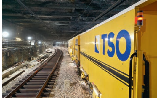
High-Impact Operation to upgrade the RER C line ▶
