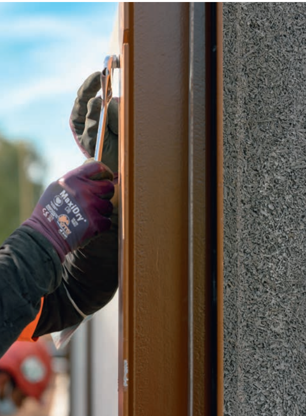
Installing acoustic screening alongside ▲ the A57
