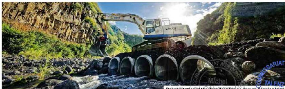
Rehabilitation of the Bras de la Plaine dam on Réunion Island
