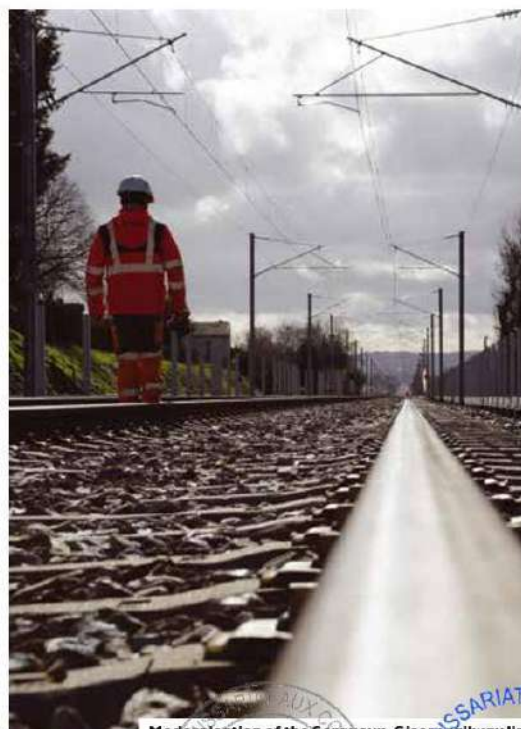
Modernisation of the Serqueux-Gisors railway line
