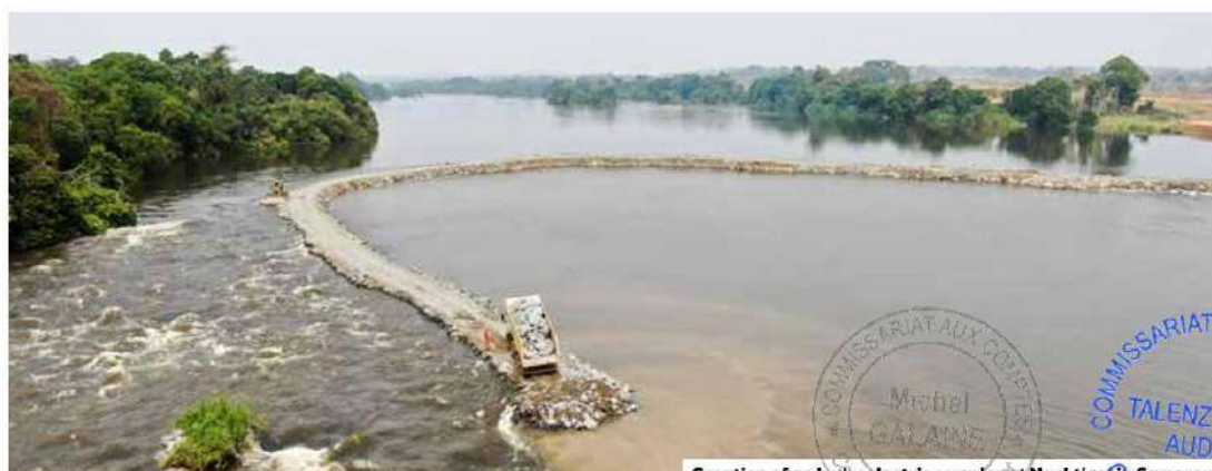
Creation of an hydroelectric complex at Nachtigal in Cameroun
