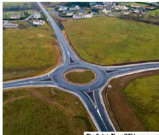
The Saint-Flour (15) bypass road
