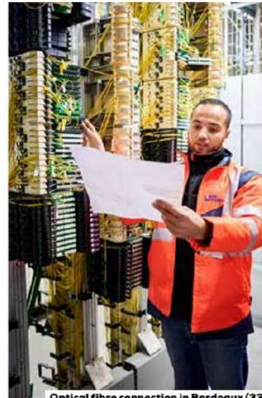
Optical fibre connection in Bordeaux (33)
