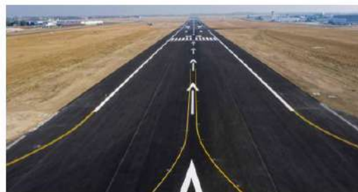
▲ Airport runway renovation Paris Le Bourget
