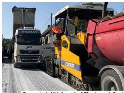
Pavement rehabilitation on the A20 motorway in Corrèze
