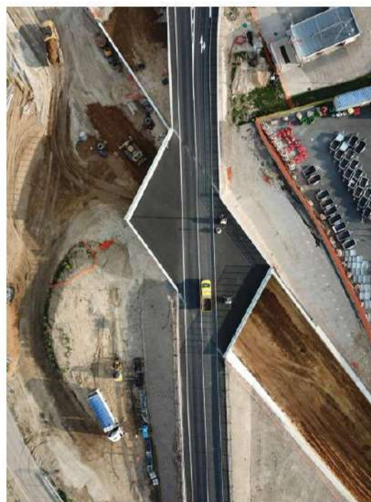
▲ Modernisation of the Serqueux-Gisors railway line (27)
