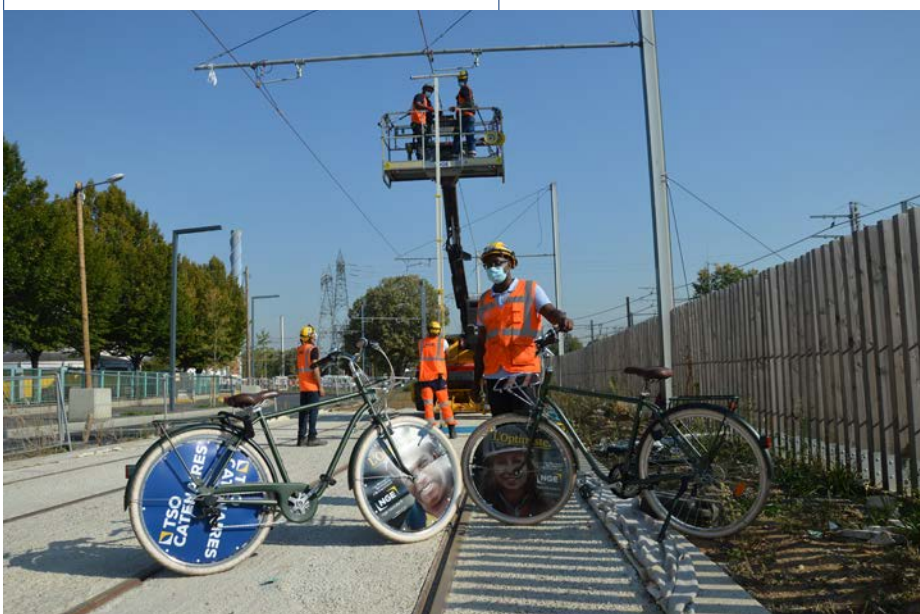
▲ The T9 Tramway worksite
