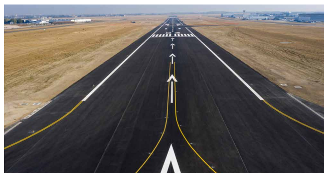
▲ Airport runway renovation Paris Le Bourget
