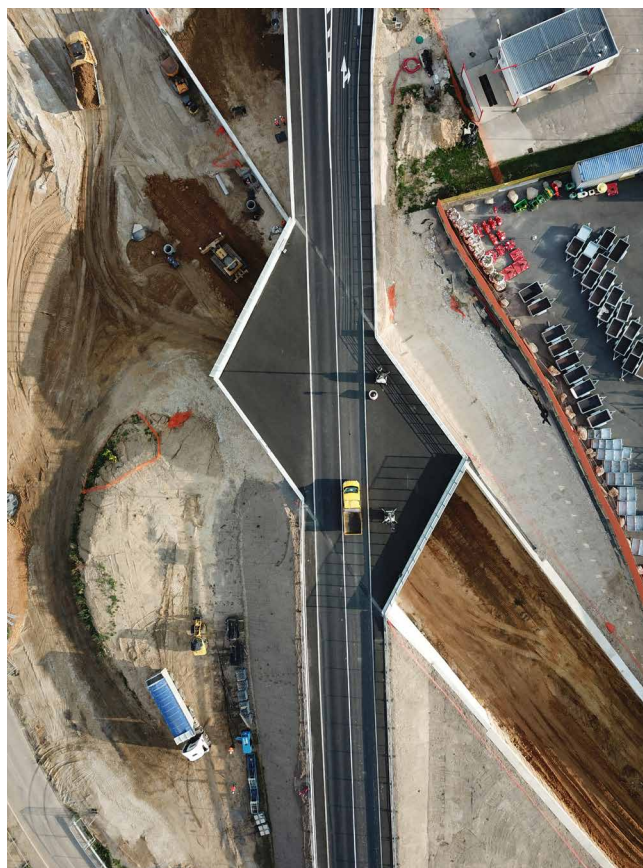
▲ Modernisation of the Serqueux-Gisors railway line (27)
